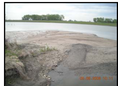
Construction site in DeKalb County that is not meeting the requirements of NPDES. Violation Notices and substantial fines from the Illinois Environmental Agency can occur if sites are found to be out of compliance.
